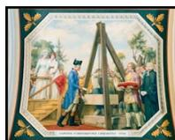
A "goat" (French: chèvre) was the common name given by the mediaeval stonemasons to the simple three-legged wooden cranes which they used to lift stones manually.
